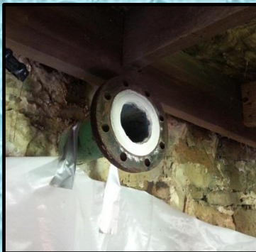
Drain pipe at pump house after Flow-Liner® Liner
