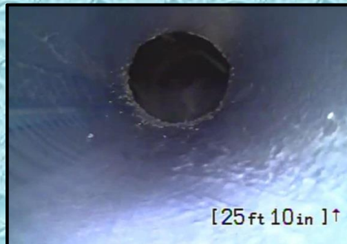
Drain pipe after Flow-Liner® Liner
