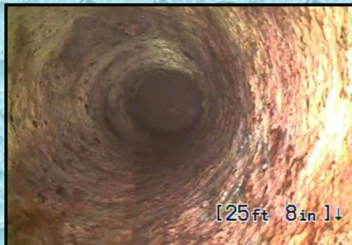
Drain pipe prior to lining
