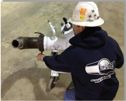
Certified Flow-Liner® Installer preparing the conduit lining inversion unit
