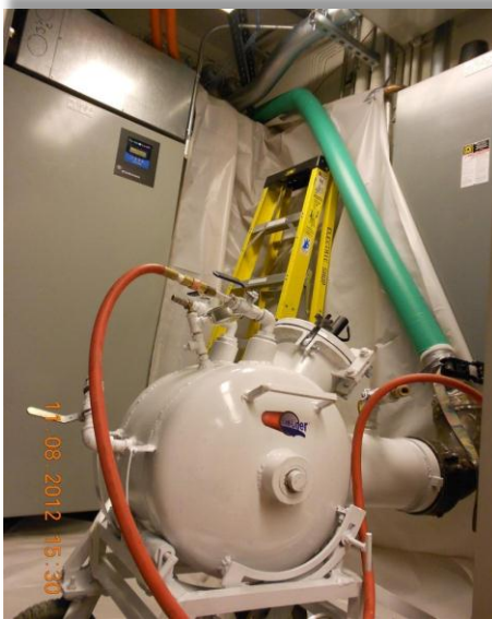
Flow-Liner® installation with the inversion unit set-up
