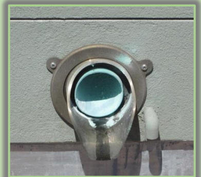
Roof drain after Flow-Liner® Installation
