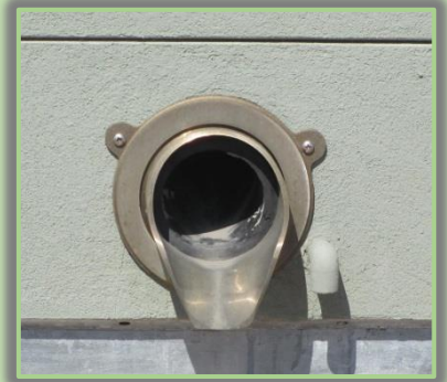
Roof drain prior to lining
