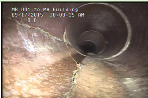
Before Flow-Liner Cured in Place Pipe Lining Installation
