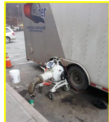
Flow-Liner equipment set-up for installation
