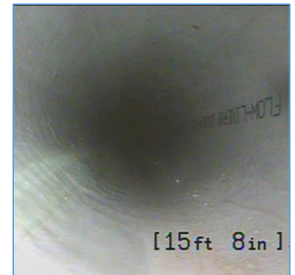
4 inch cast iron after Flow-Liner® installed
