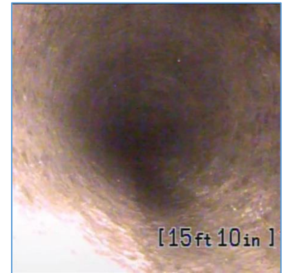
4 inch cast iron pipe before lining
