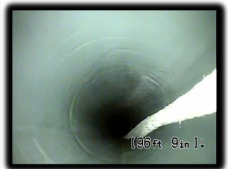
10 inch fiberglass pipe after Flow-Liner® installed
