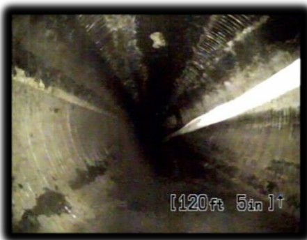
10 inch fiberglass pipe prior to lining
