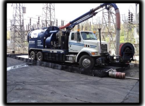
Pipe Cleaning Equipment Set-up
