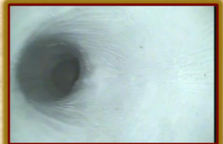
Cast iron pipe after Flow-Liner® installed
