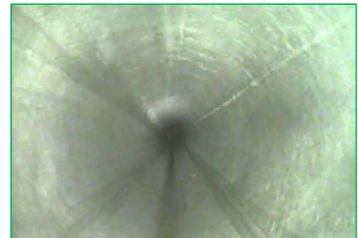
After Flow-Liner ® Installation
