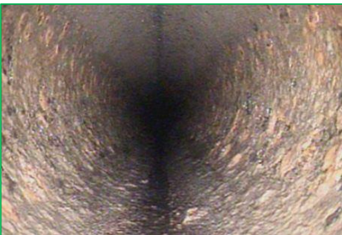
Before Flow-Liner ® Installation
