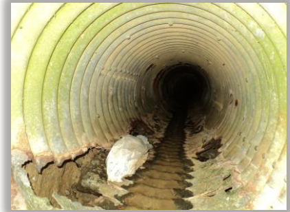
Condition of culvert before lining
