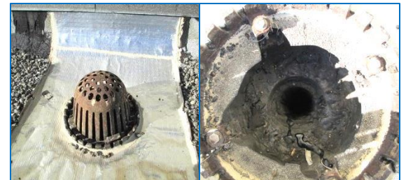
Roof drain before Flow-Liner® Installation
