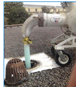
Flow-Liner® Inversion Installation in progress
