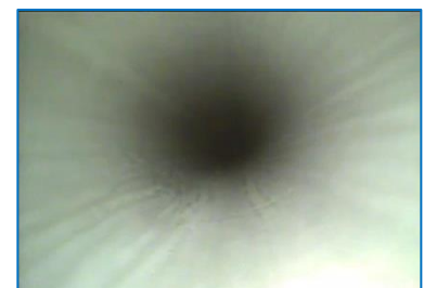
Roof drain after Flow-Liner® installation
